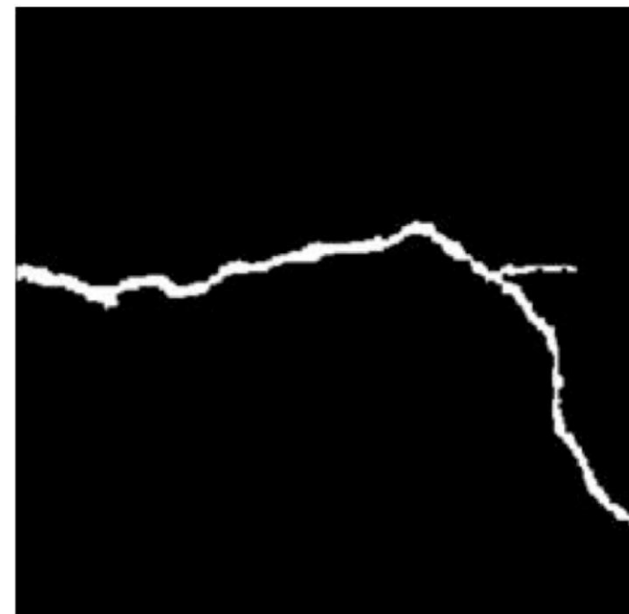
Crack detection image
